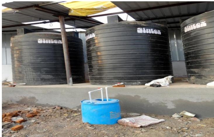
**Figure 2: Vermi-bio-filters with buffer tank**
