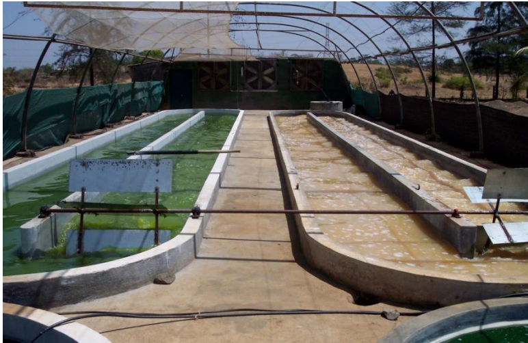
Figure 2: Open channel raceway ponds for BRC's IMAET biotechnology treatment
